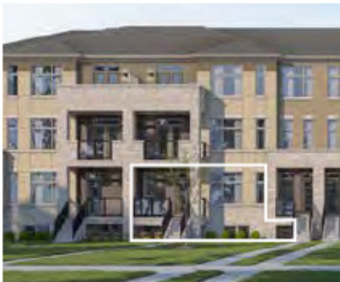
FRONT, Interior Unit
